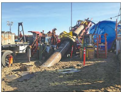
Casing for the desal test well being drilled in Marina heads underground at the requisite 19 degree angle. Construction started a few days after Christmas.
